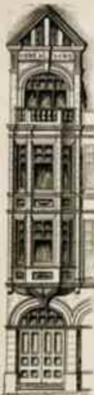
ENTRANCE: BLACKFRIARS STREET MANCHESTER.
